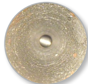
Deposits in pipe
