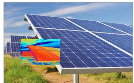
Photovoltaic thermography from the air
