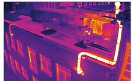
Temperature monitoring for building thermography
