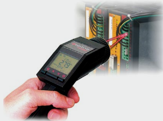
Detailed infrared temperature measurement of an electric control with the help of the installed close focus optics for 1 mm ranges of the LS
