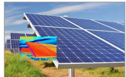
Photovoltaic thermography from the air
